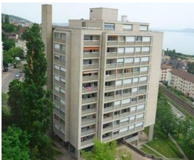
Fig. 3: Building image (current status).
